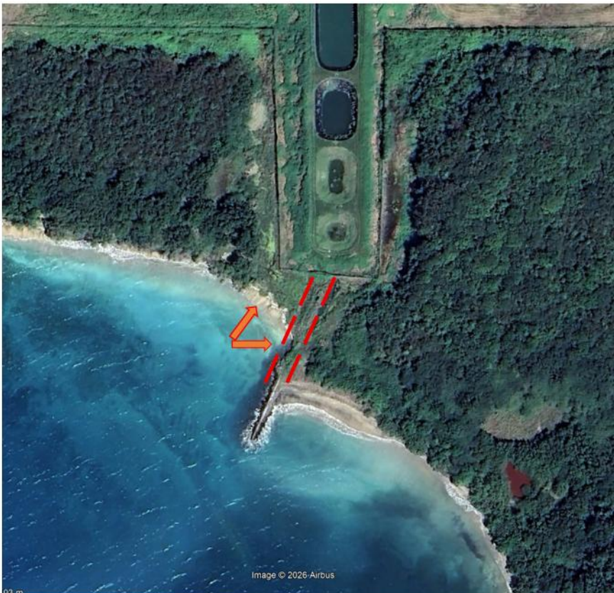
Figure 2: Top: Airport region WLR (m/yr) between 2010 and 2025. Bottom: Google Earth images of the outfall / groyne structure, to the south of Maurice Bishop Airport. Arrows mark eroding frontage that may affect the structure and ultimately the ponds, and dashed red lines mark a linear ridge between the groyne/outfall and the ponds, which is possibly a buried pipeline.
